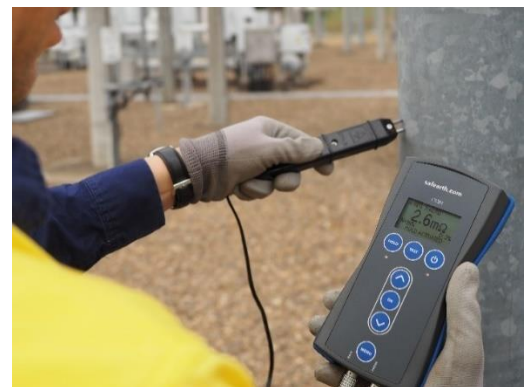
Continuity testing using the Safearth CS3 Site Continuity Meter
